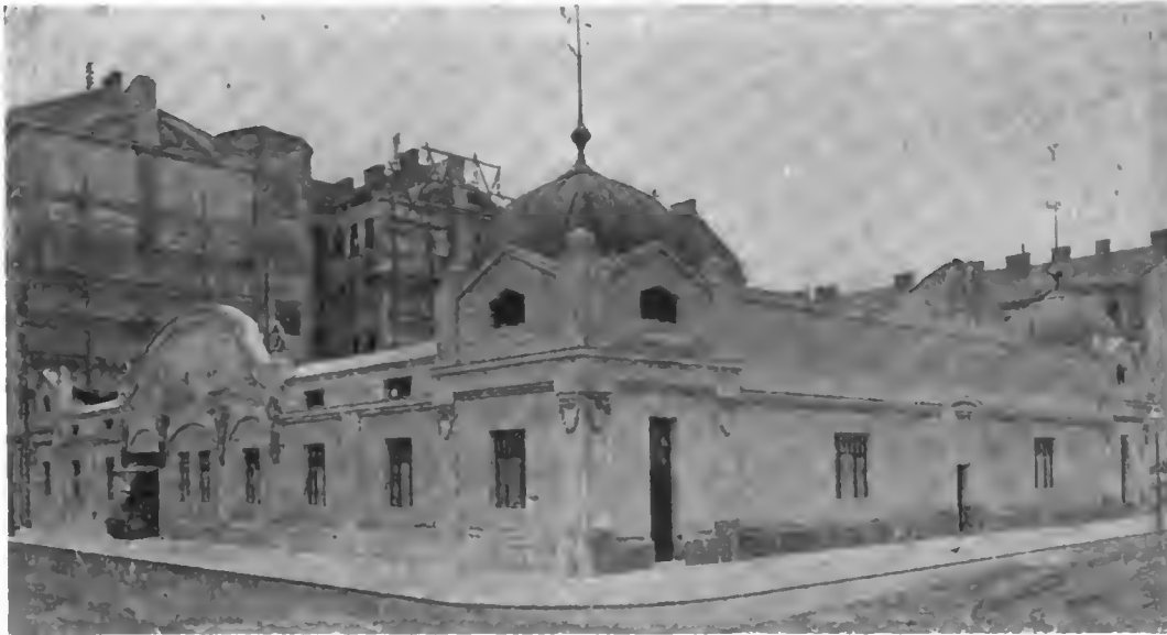
Where the electric mail vans are garaged in Vienna. The building is 131 by 102 feet, of one story and basement, and fronts on three streets. The interior, together with the idea of stalls for the cars, is illustrated below
